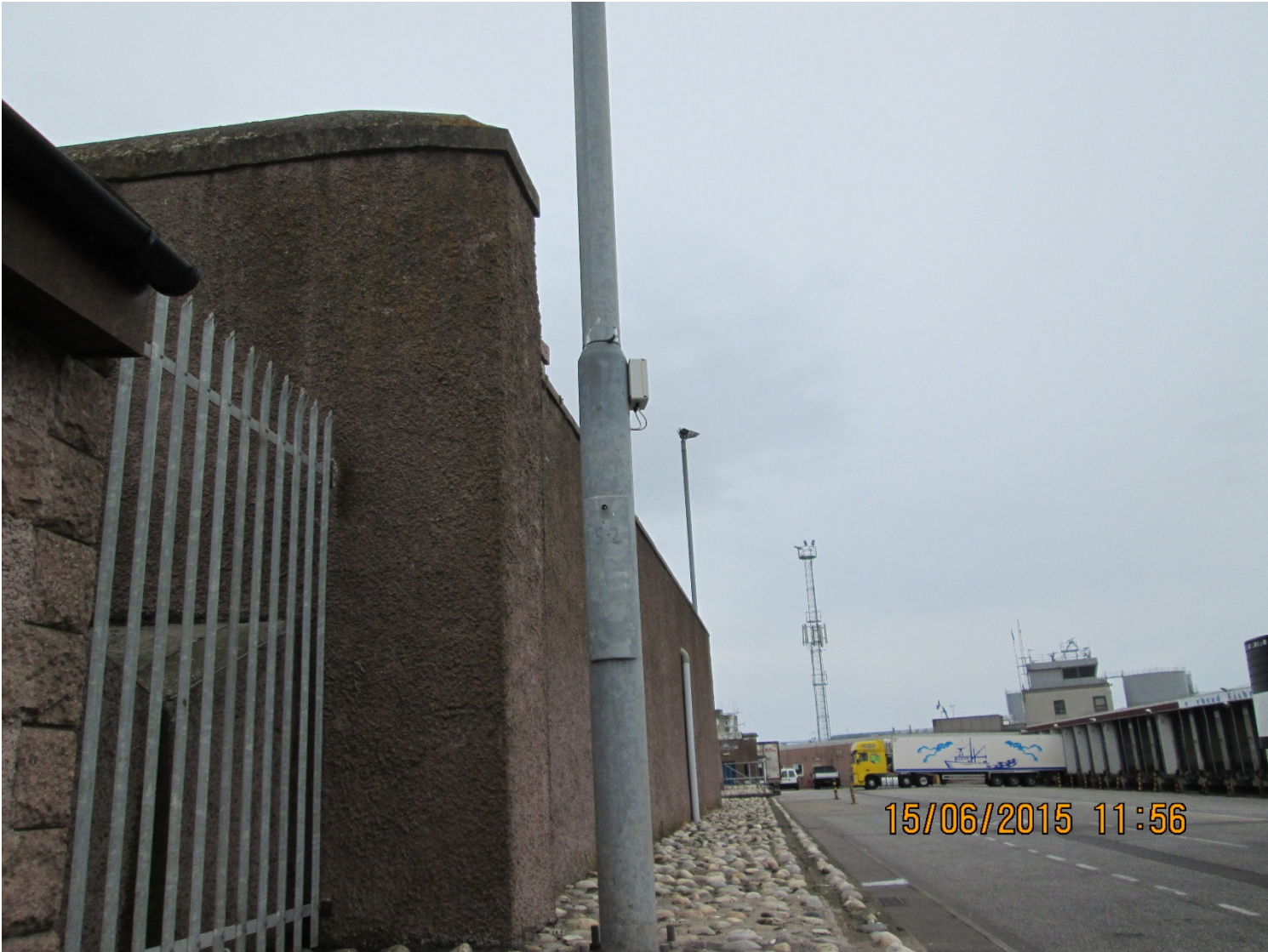
Figure D.3 Fishmarket: View toward lorry bay at fishmarket
