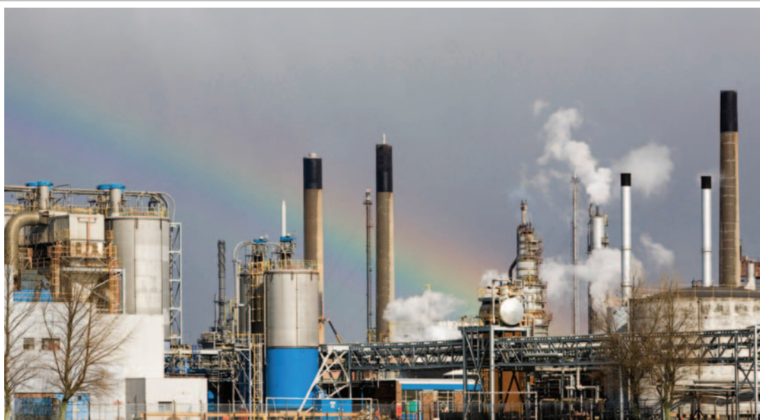
Figure 3.2 Grangemouth Refinery after a storm. Industry remains an important source of air pollution in some parts of Scotland
