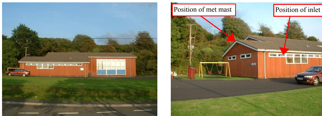
Figure 2.2: Building in which the monitoring equipment was housed. The equipment was located in the left hand portion of the building.
