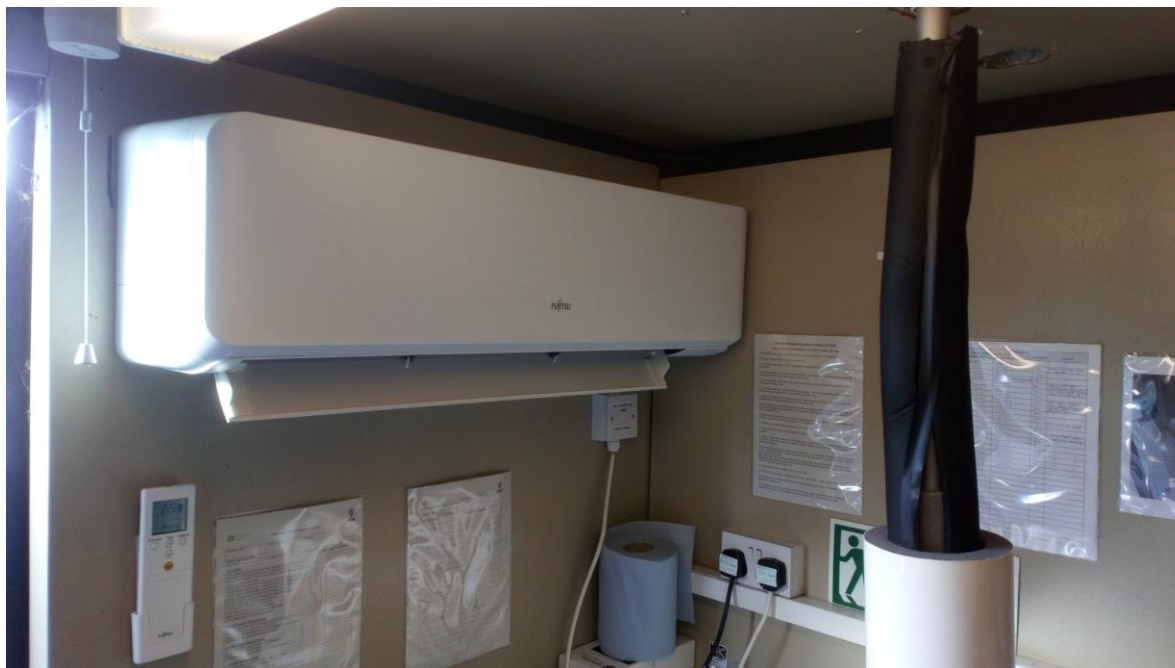
Photo 5 New Air Conditioning Units Installed at the Grangemouth AURN Site
