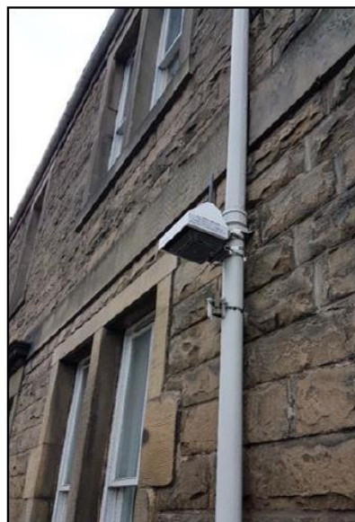
Appin Crescent West AQMesh Sensor (co-located with triplicate diffusion tubes Appin Crescent 6A, B, C)
