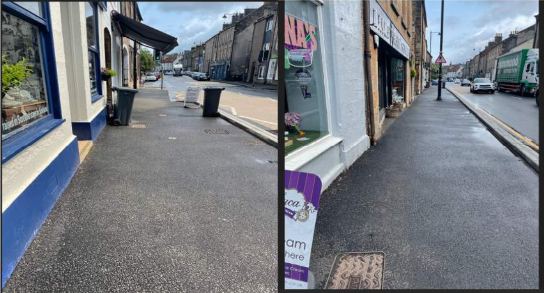
Photo 2.1 – Example of permanent pavement widening in West Lothian on Linlithgow High Street completed in 2024.
